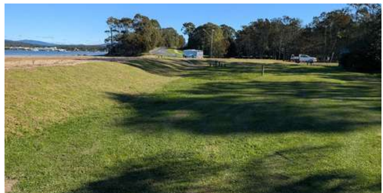
Surfside levee complete
