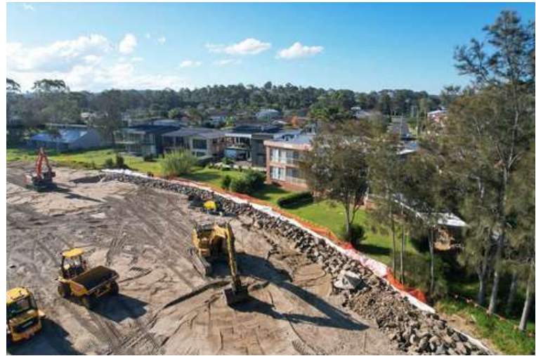
2,700 tonnes of rock used to build the levee.
