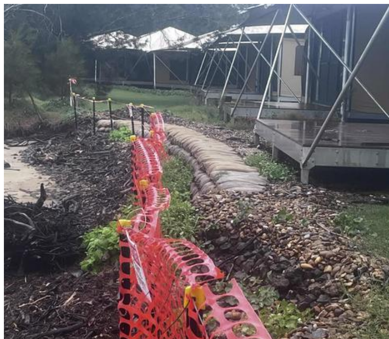
The sandbagged Myamba Eco Resort yesterday.
