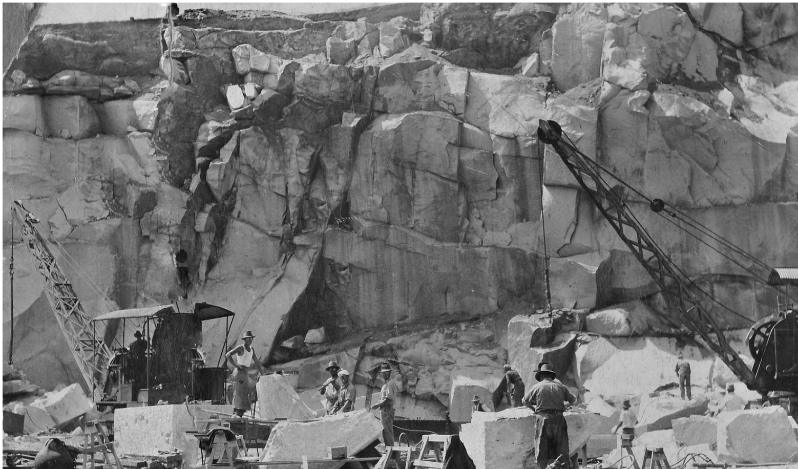
Cranes working at the quarry face
