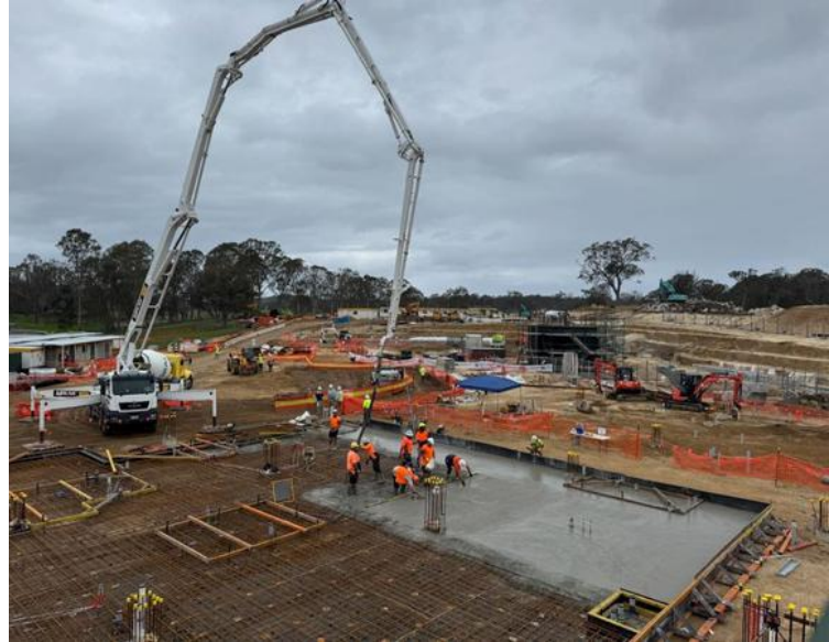
Concrete slab for the first paediatric department in the region.
