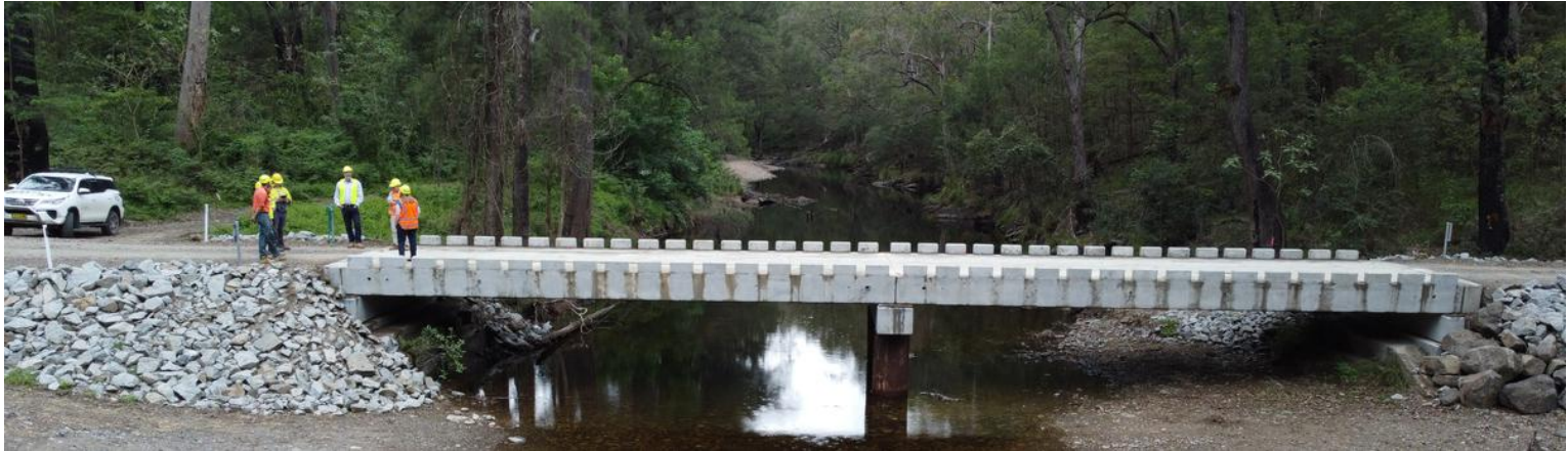
Forestry Corporation staff from Southern Region Forest Infrastructure Repair Program (FIRP) with Minister Moriarty on Lyons Road Bridge north-west of Batemans Bay
