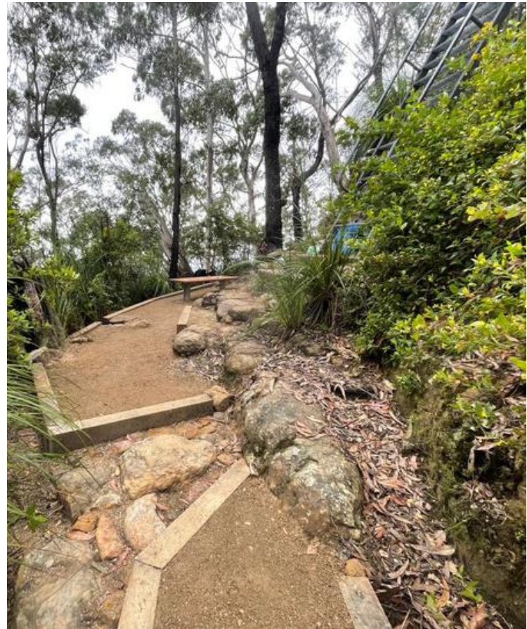
After pad construction and new chair
