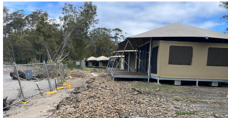
Beach erosion at Surfside
