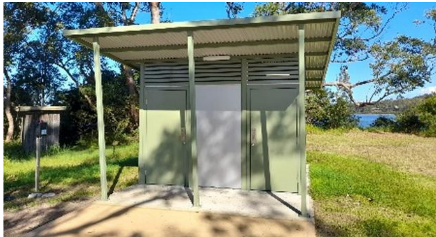
A modular toilet block
