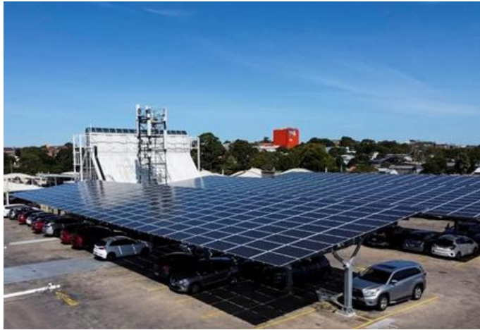
SHASA representative met with Dr Michael Holland this week to discuss solar for the new hospital. Example above.
