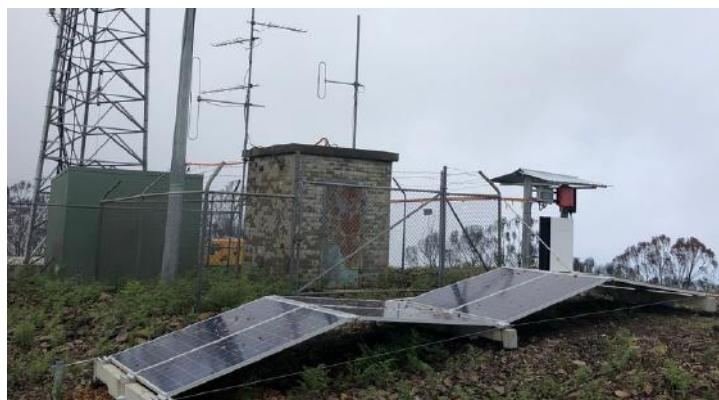
'Peak Alone SAPS': The stand-alone power system and communications tower at Peak Alone near Cobargo. Photo: supplied Essential Energy.
