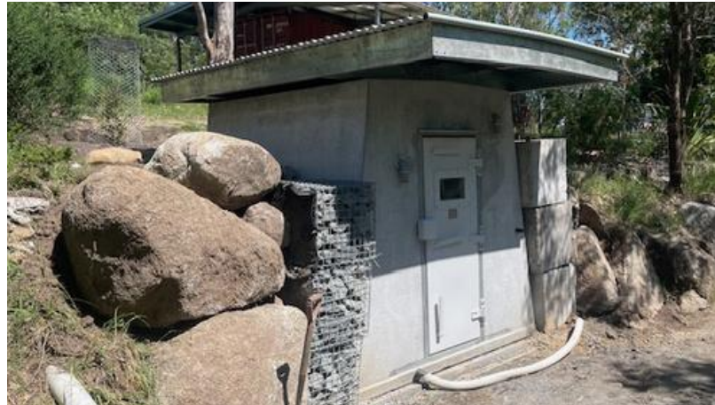
The bunker built into bank.
