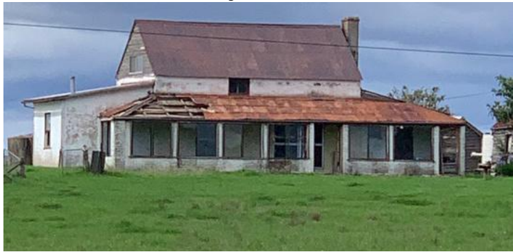
One for a keen renovator: Shannon View on Larrys Mountain Road.
